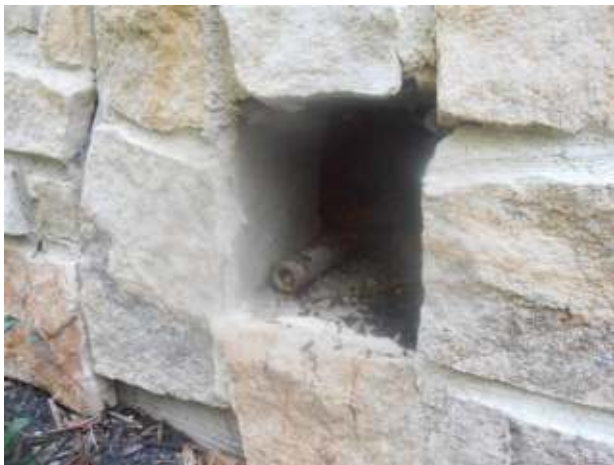
The open exterior fireplace ash pit needs to be covered.
